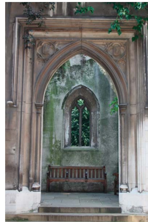
The ruined church of St Dunstan's in the East, now a City garden.
